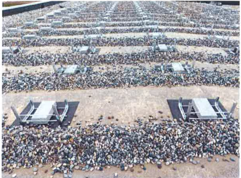
In Progress Ballast Bay Installation
