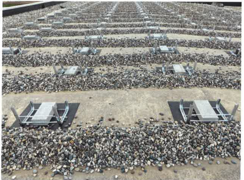
In Progress Ballast Bay Installation
