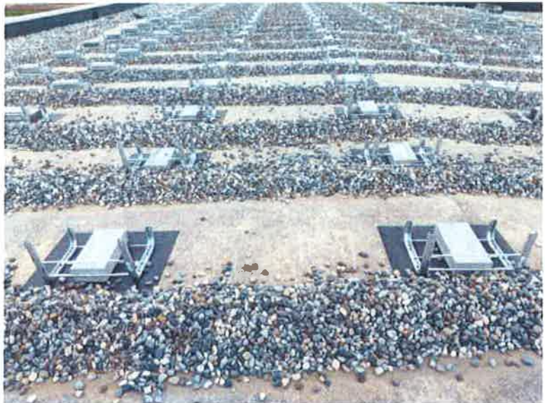
In Progress Ballast Bay Installation
